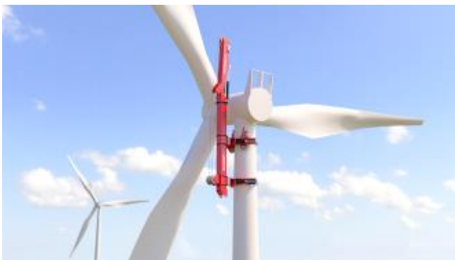
WTM 100 at elevation, ready to start turbine service.
