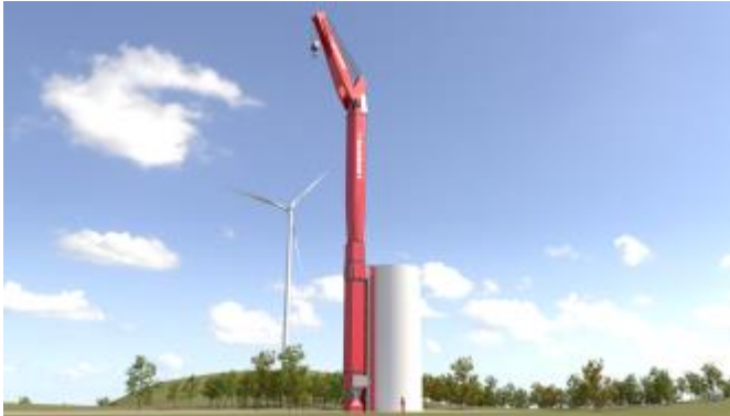
The WTA 250 ready to lift the 2 nd tower section.
