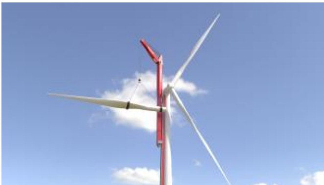
Installation of a turbine blade using the WTA 250.
