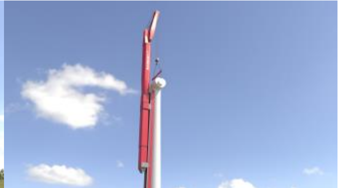
Installing the nacelle with the WTA 250.
