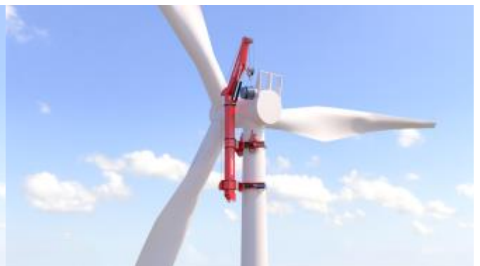
Replacing a generator with the WTM 100.
