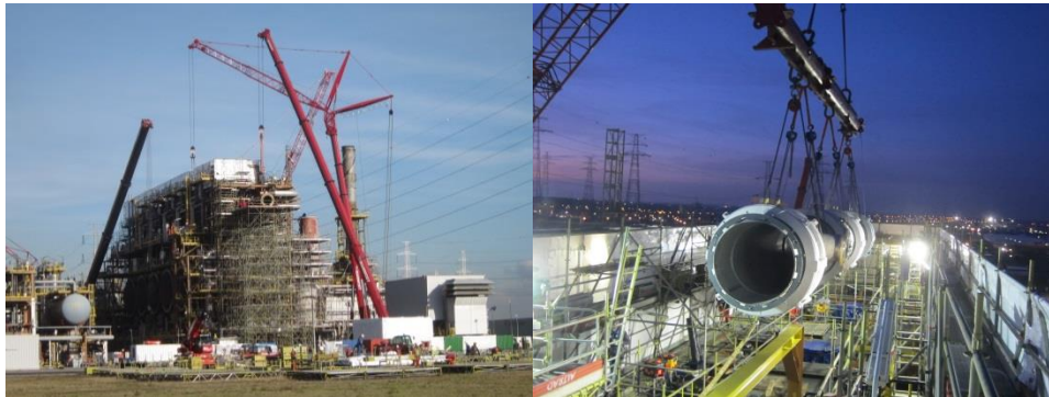
Photos: Turnaround project and exchange of header Copyright 2014 Borealis Kallo
